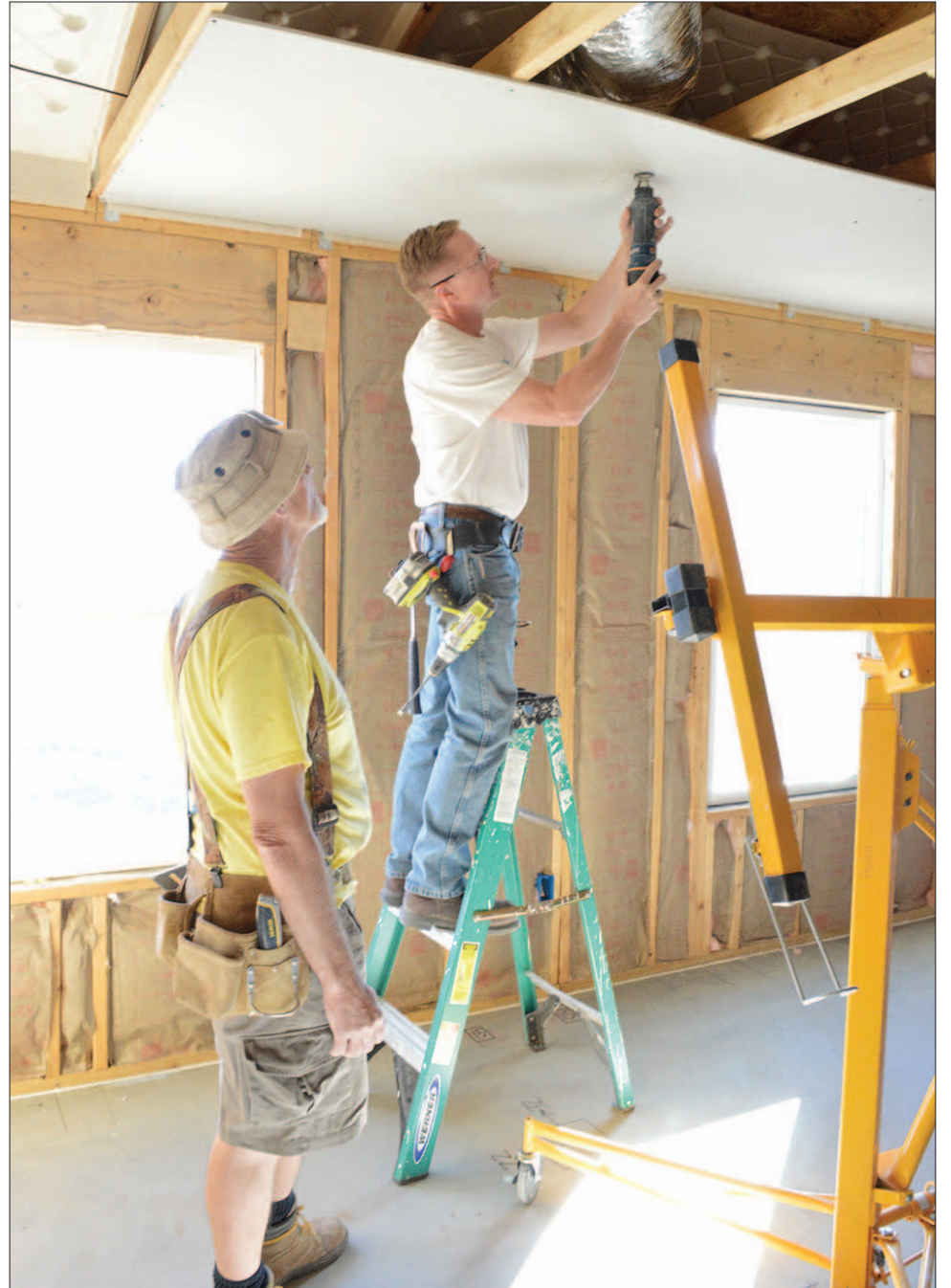
MVHFH Construction Superintendent Pete Pemberton shows a volunteer how to properly cut a hole for a vent in sheetrock Tuesday, Oct. 1.
