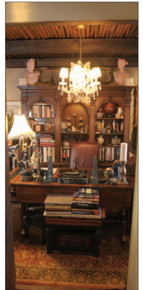
Latillas cover the office ceiling.
