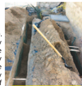
400' Copper Tubing Install
