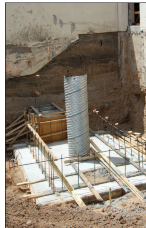
The beginnings of a two-story elevator shaft
