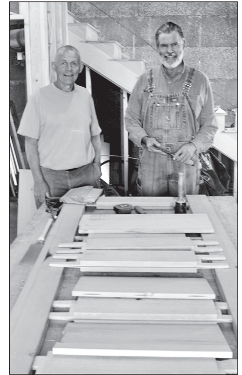
Las Cruces Bulletin photo by Beth Sitzler Watson MacKinnon and John Hyndman are working on the new front doors of Phillips Chapel CME, one of the last items needed for the restoration project of the 100-plus-year-old adobe church.
