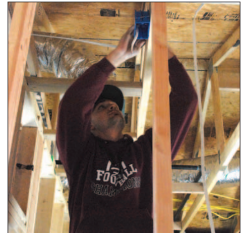
First-year apprentice Justin Taylor participates in the class, which included running outlets, installing the wiring for lights and smoke detectors and installing boxes for light fixtures.
