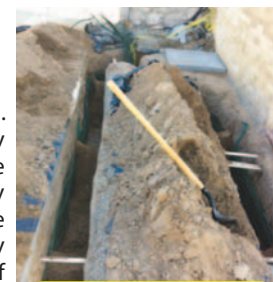
400' Copper Tubing Install
