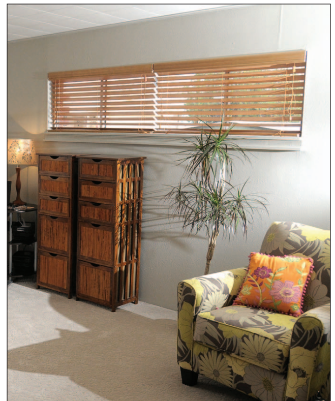
Clerestory windows were used for light and privacy.
