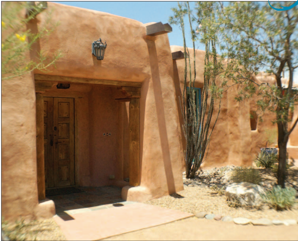
The adobe home at 3205 Linden Ave. was built as a one-bedroom abode in 1901.
