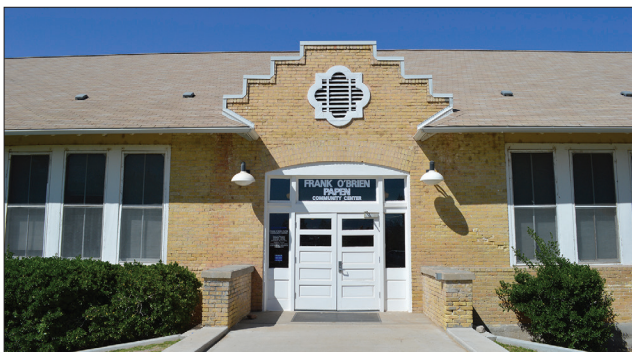
The Frank O'Brien Papan Community Center, built in 1907, was recently discovered to be designed by Henry Trost, who helped shape El Paso and much of southern New Mexico in the 20th century.
