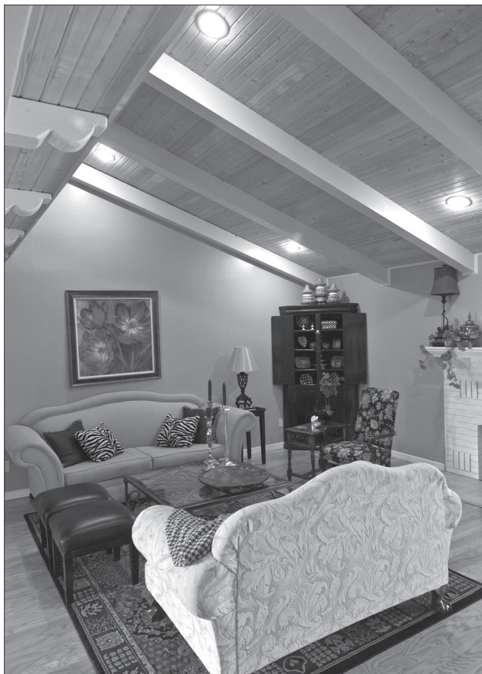
Large beams and tongue-and-groove planks cover the vaulted living room ceiling.
