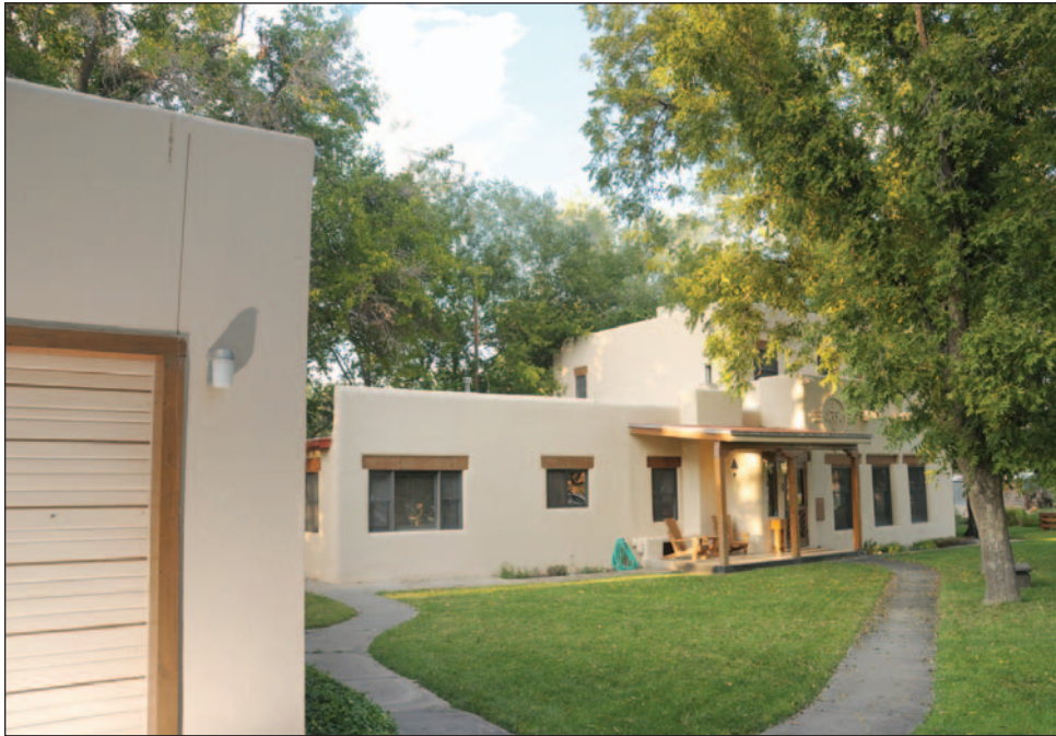
The home at 700 Watson Lane was originally built as a one-bedroom home in the early 1940s. It now spans 3,000 square feet.
