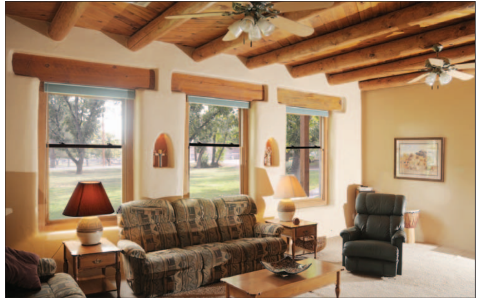
A living room built out of rammed earth was added to the home. The room includes vigas and a tongue-and-groove pattern on the ceiling.
