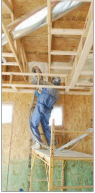
Las Cruces Bulletin photos by Beth Sitzler **Oscar Covos of Ontiveros** Insulation installs the spray foam insulation on the ceiling, a process that will take two days to complete.
