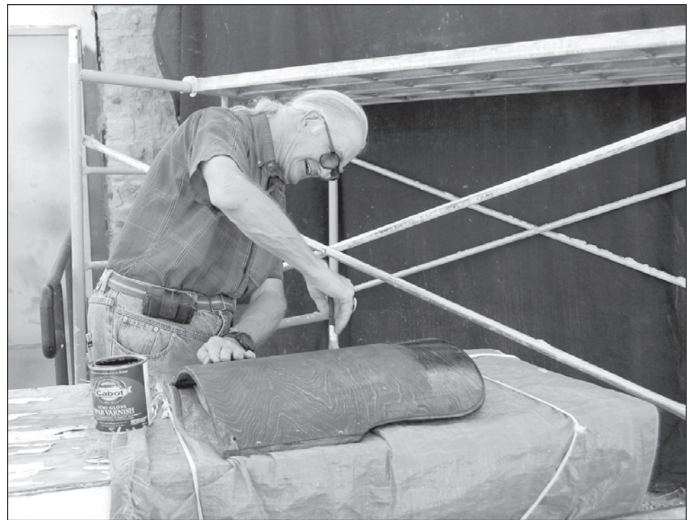
Bobby Hutson adds varnish to the theater seats at Phillips Chapel CME Church Wednesday, Aug. 29. Due to age, the seats, originally built in the 1930s for the Del Rio Theatre, had begun to split and become loose.
