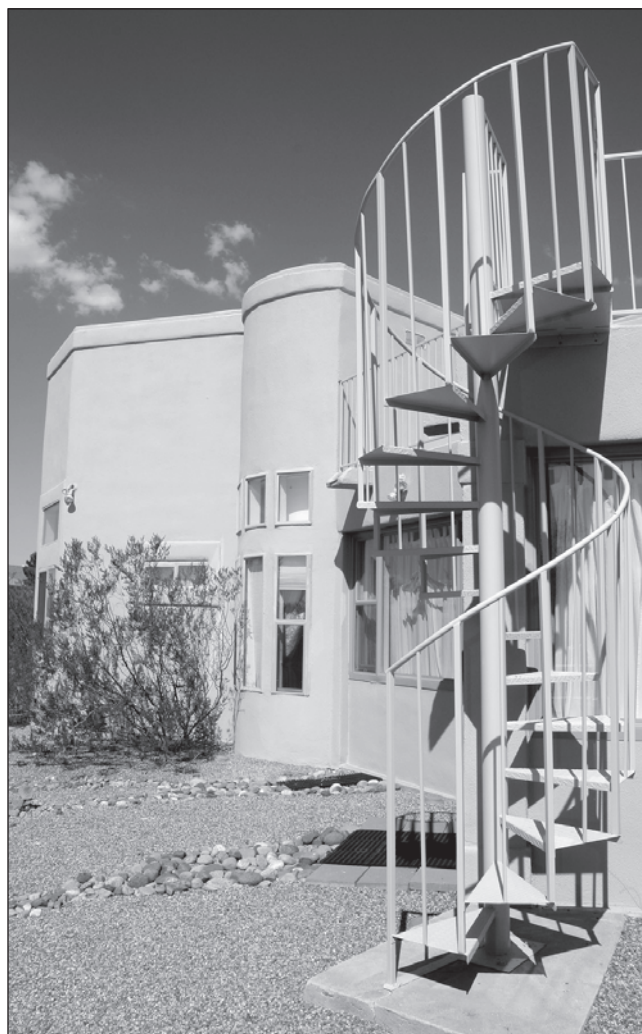
A spiral staircase leads to a veranda on the roof.
