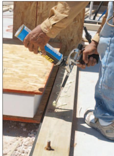
**Before the structural insulated panel is put in place, expanding foam is applied by Muñoz.**
