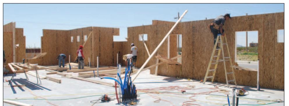
The NetSolar Construction home at 3602 San Clemente has begun to take shape. Using structural insulated panels, a vapor barrier and a tankless water heater are some of the ways the home is being built to LEED platinum certification.
