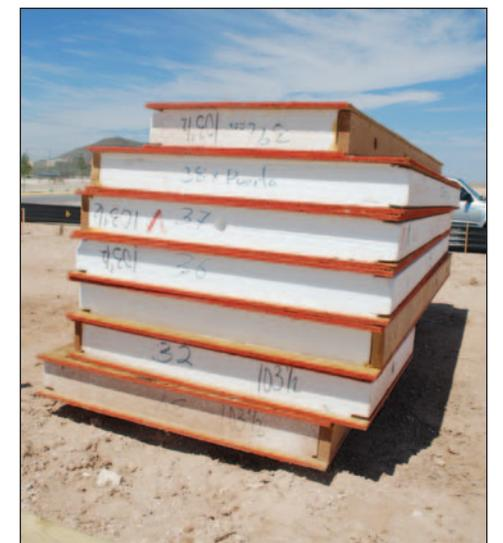
**Numbers are written on the SIPs that match the floor plan to ensure each is placed exactly where it's supposed to be.**
