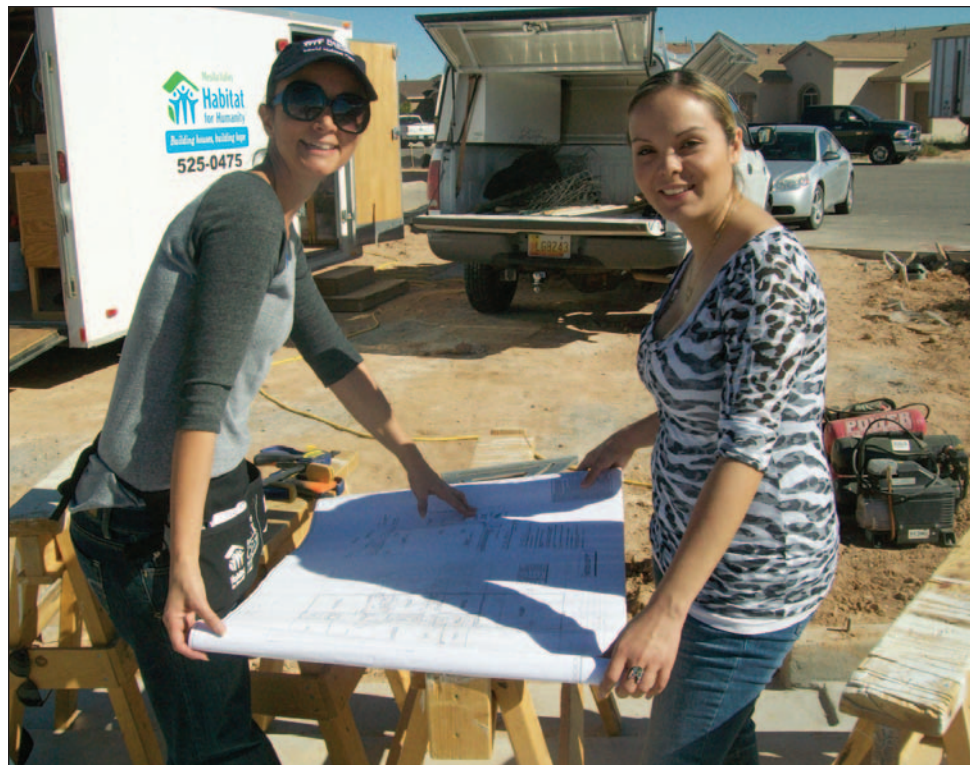
Mesilla Valley Habitat for Humanity Executive Director Marie Schwartz and home recipient Anais Muñoz look over the plans of Muñoz's future home, now under construction. After joining MVHFH in 2009 as the development officer, Schwartz took over the executive director position on Nov. 1.
