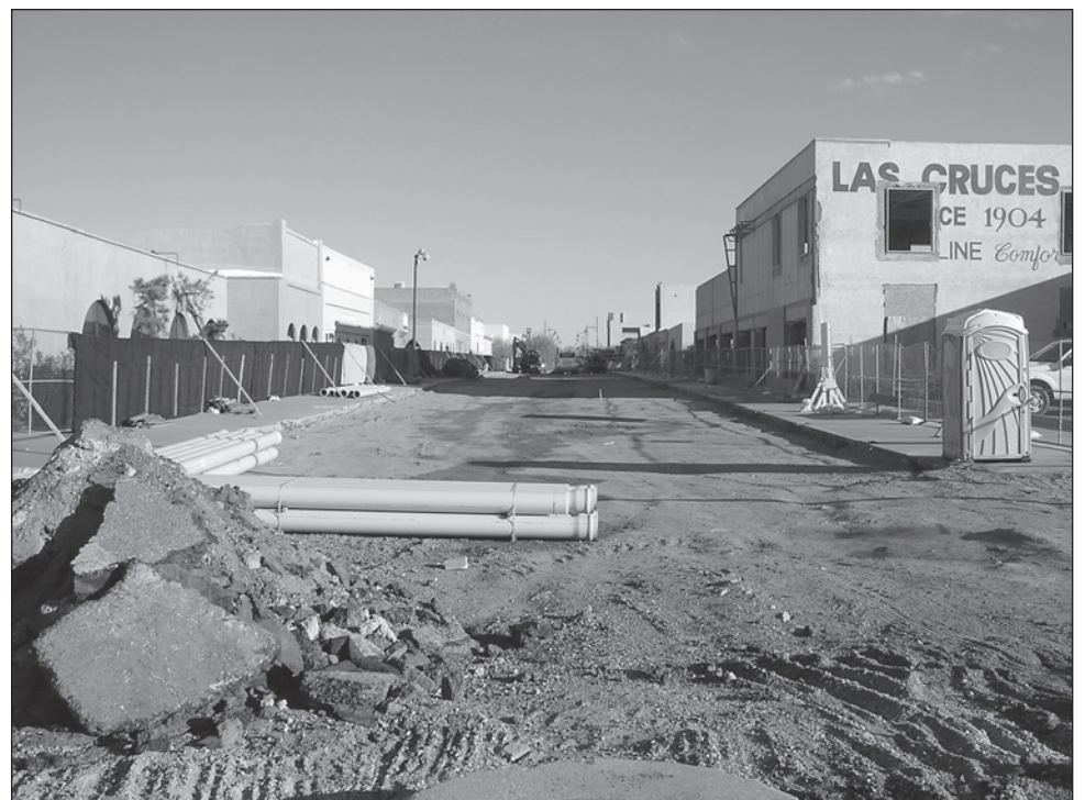
The street is prepared for pipe installation.
