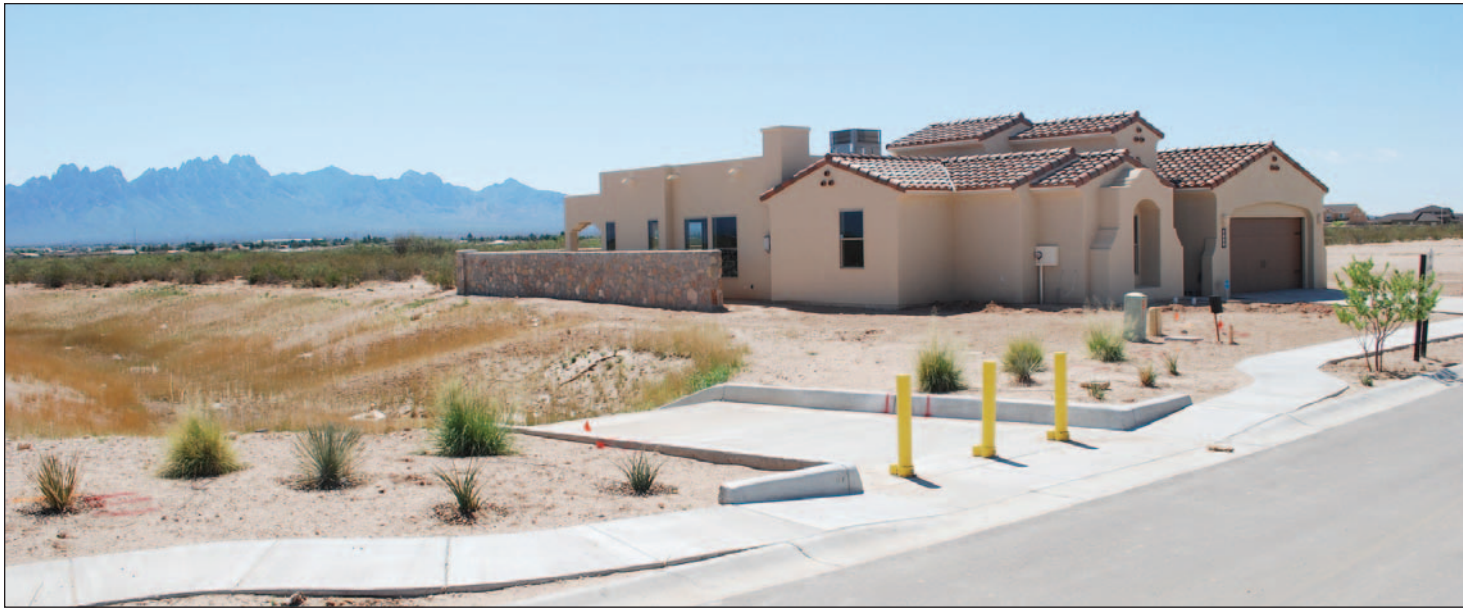
As part of the requirements to earn National Association of Home Builders green subdivision certification, the storm water system of Metro Verde was seeded and planted to prevent erosion. Also, discarded plant material from the area was incorporated into the arroyos.
