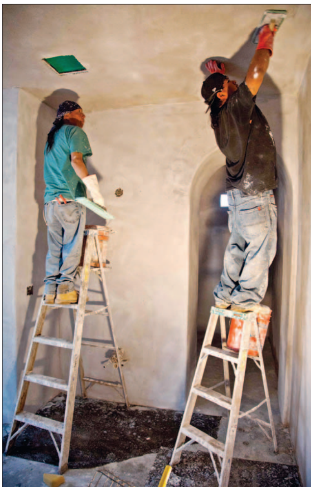
Eric and Todd Calabaza apply lime plaster to a wall.
