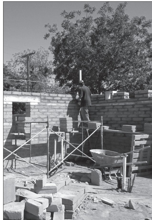
Adobe bricks from the Mesilla Valley were used to create the addition, which expanded the square footage to 2,300.
