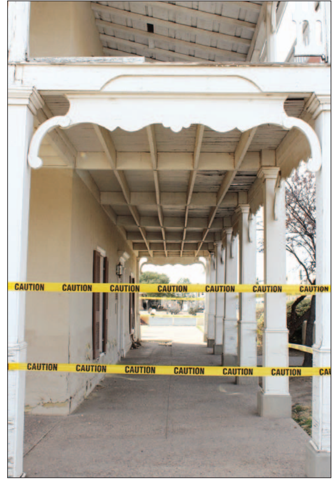
The Nestor Armijo House, 150 E. Lohman Ave., is currently being rehabilitated and will be the future home of the Greater Las Cruces Chamber of Commerce.
