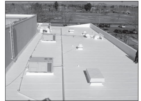
The above photo shows an original roof needing repair. Below, with elastomeric, the roof is now energy efficient.
