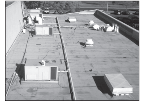
The above photo shows an original roof needing repair. Below, with elastomeric, the roof is now energy efficient.
