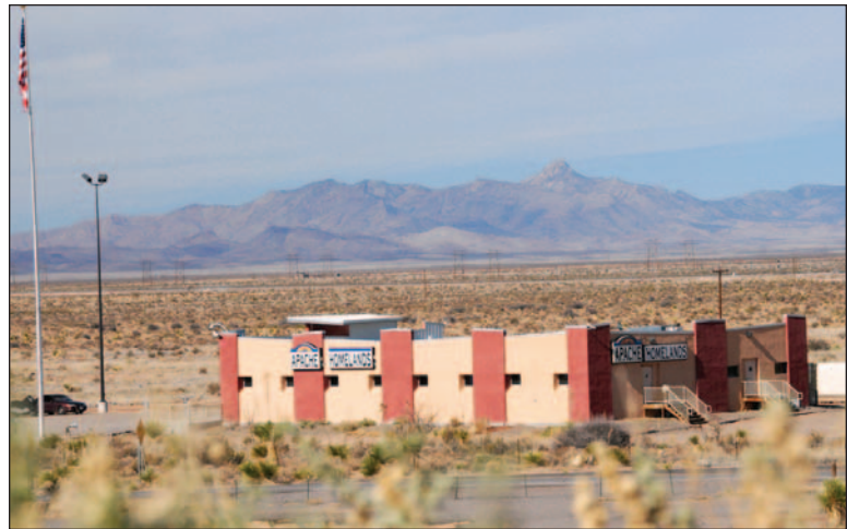
This is the Apache Homelands Casino building in Akela Flats, which was built in anticipation of the tribe someday getting approval for American Indian gaming activities.
