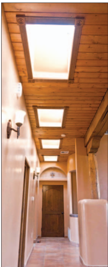
Planks line a ceiling and trim surrounds the skylights.
