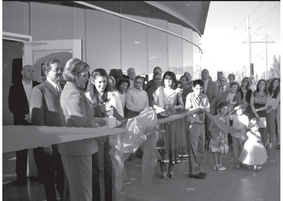
Las Cruces Bulletin photo Gov. Susana Martinez and Shinye Nattakom cut the ribbon on the new Green Offices building on Roadrunner Parkway Tuesday, April 24. The building has multiple features focusing on sustainability, including water-use reduction, a 36-kilowatt solar electric system, heat-rejecting glass and low energy use air conditioning units.
