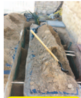
400' Copper Tubing Install
