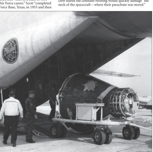
The battered Gemini VIII capsule is loaded onto a cargo jet for return to NASA and a study of why it malfunctioned.
