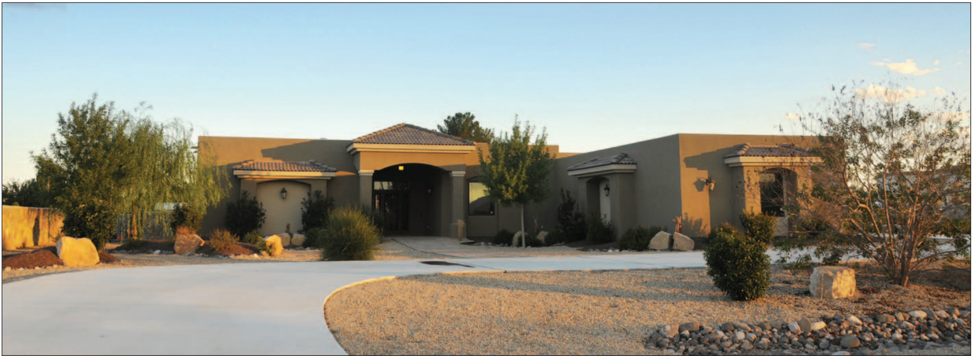
Built in 2009 by Ned Tutor, the home at 1869 River Court features 3,260 square feet of space on a 1.03-acre lot off Taylor Road in the Mesilla Valley.
