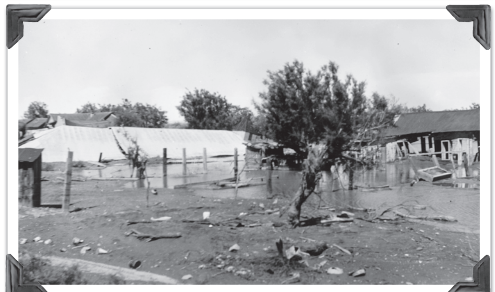
Photo reproduced courtesy of the New Mexico State University Library Rio Grande Historical Collection In the top photograph, dated May 16, 1937, the Catholic church at San Marcial remains standing, but in the bottom photograph, dated May 31, 1937, only the tin roof and steeple remain after the building's adobe walls disintegrated during the floods that devastated San Marcial in that year.
