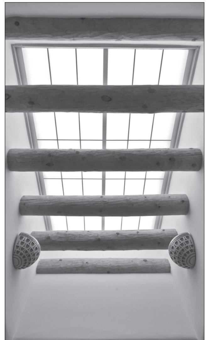
Skylights add natural light throughout the home.
