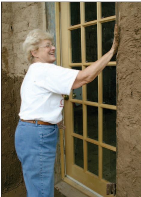
MVP volunteer Sara Orton applies mud plaster the old-fashioned way to a Mesilla building.
