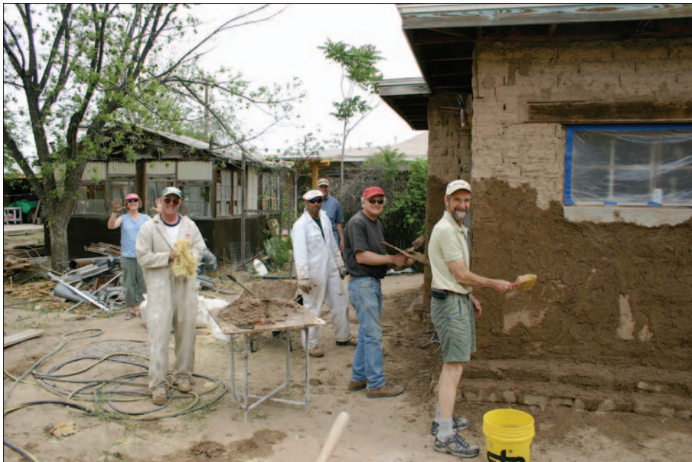
Mesilla Valley Preservation Inc. board members and volunteers get their hands dirty during a mud plaster workshop held by master plasterer Larry Limon (third from the right) at a Mesilla casita.
