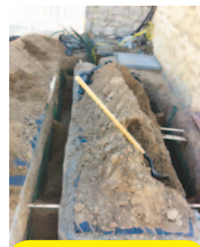
400' Copper Tubing Install
