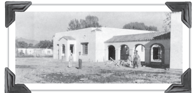
Construction underway at the current site
