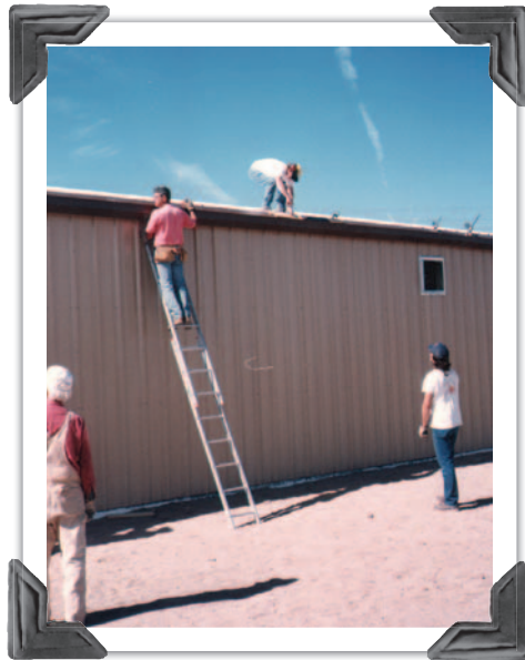
In 1996, MVHFH moved away from New Mexico State University and into its office on Santa Fe Street. The location also used to house the ReStore, which is now off Main Street.
