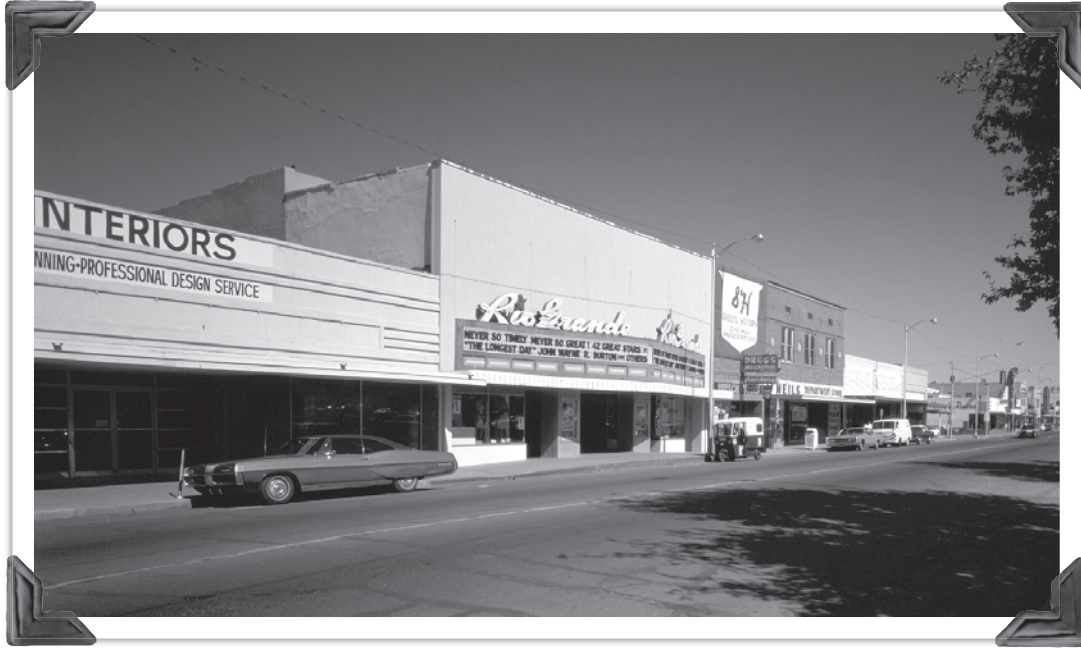
The Rio Grande Theatre was covered by a false front in this photograph on Main Street. "The Longest Day," listed on the marquee, dates from 1962, but the '67 Pontiac Bonneville shows the film was not in its first run when this photo was taken. In that era, shoppers could get Green Stamps with their prescriptions, and mail was delivered using a three-wheeled vehicle called a "Mailster."
