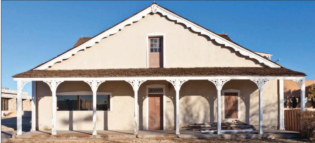
A two-story addition was constructed onto the Nestor Armijo House in 1877. It was uncommon for homes in the area to feature a pitched roof during that time.
