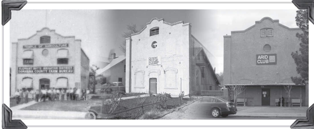
Unlike many historic buildings in Las Cruces, the structure at 334 W. Griggs Ave. has escaped the wrecking ball. The building was once called the "Temple of Agriculture," and housed the Elephant Butte Irrigation District and the Doña Ana County Farm Bureau. Later, it was the Gospel Rescue Mission, and today, the structure is the Arid Club, an alcoholism treatment center.
