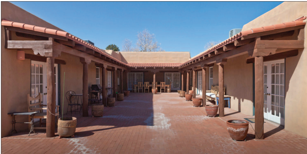
The hacienda at 6612 Vista Hermosa features a traditional U-shape design with a courtyard at the center.
