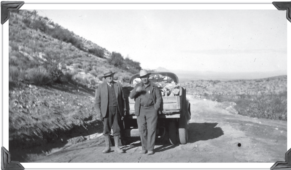
Two unidentified gentlemen pause with a truckload of dirt and rock near Organ, in this undated photograph by Organ merchant Louis B. Bentley.
