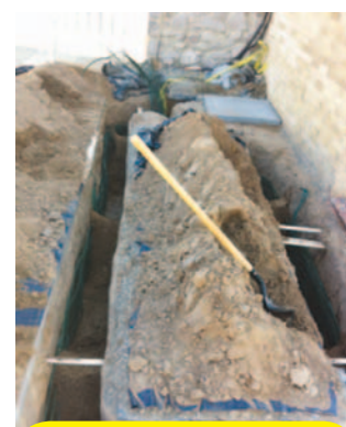
400' Copper Tubing Install
