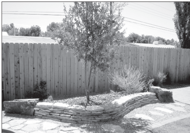
This rock ledge is an example of work done by Majestic View Construction & Landscaping.
