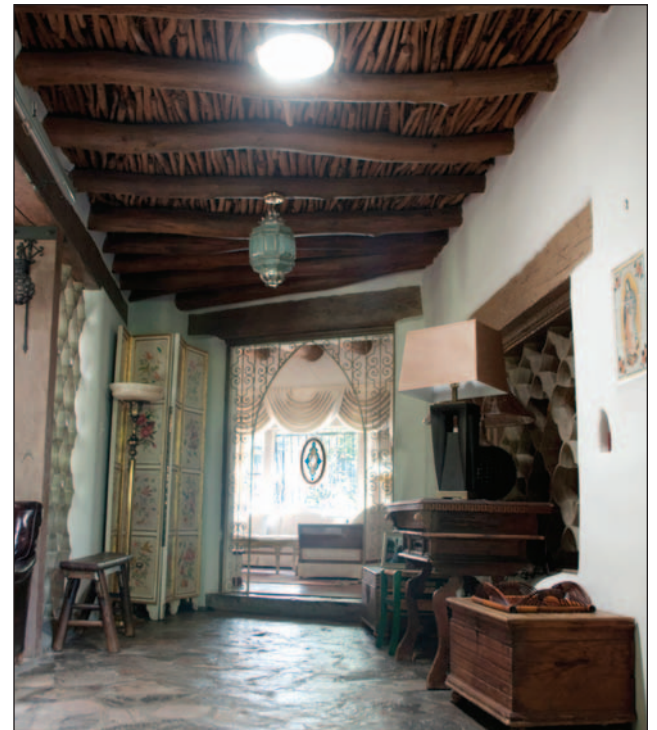
Latillas, vigas and rocks with fossils fill a hallway.
