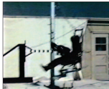
These United State Air Force images are from a film taken in September 1956, showing Dr. John Paul Stapp during a Swing Seat test that gauged the effectiveness of seat belts. A cable pulled Stapp back, and at release he swung forward until the cable jerked him – painfully – to a stop.
