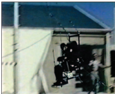
These United State Air Force images are from a film taken in September 1956, showing Dr. John Paul Stapp during a Swing Seat test that gauged the effectiveness of seat belts. A cable pulled Stapp back, and at release he swung forward until the cable jerked him – painfully – to a stop.
