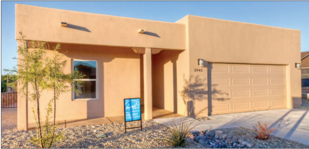
The home at 3945 Sombra Morada is Energy Star certified and has a HERs rating of 65.
