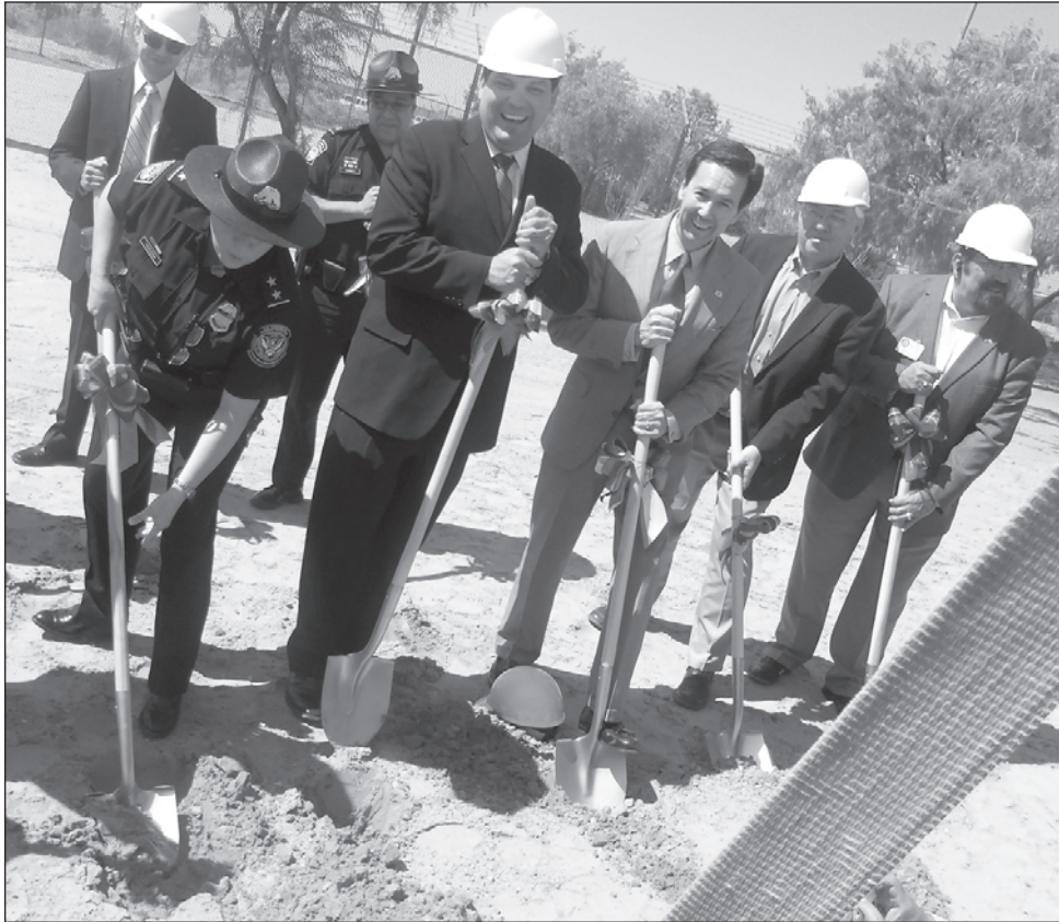
Ana Hinojosa, director of field operations-El Paso for the U.S. Customs and Border Protection Department of Homeland Security, scoops another pile of dirt while J.D. Salinas, regional administrator for the U.S. General Services Administration, and Secretary of Economic Development Jon Barela share a laugh during the Santa Teresa Port of Entry groundbreaking ceremony Thursday, July 7.
