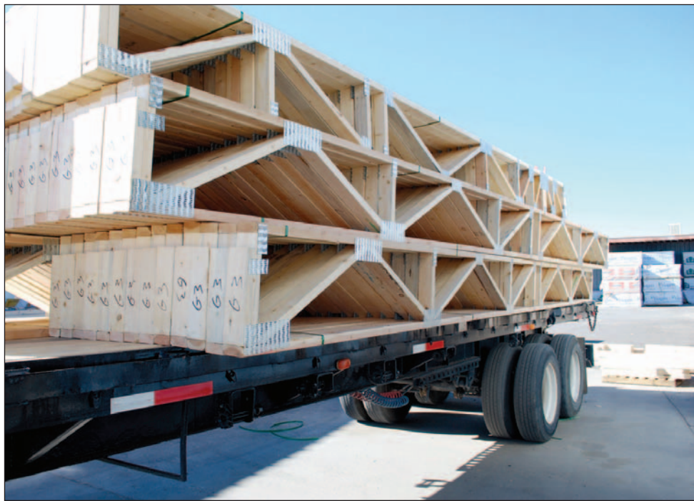
Floor trusses for the second story of an apartment building are loaded and ready to be hauled off the 7-acre property.
