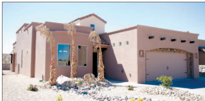
Ricardo Rasura of Rasura Custom Homes completed this Tuscan abode at 4140 La Purisima in February. The builder works to include fine detail in all of his homes, no matter the price range.
