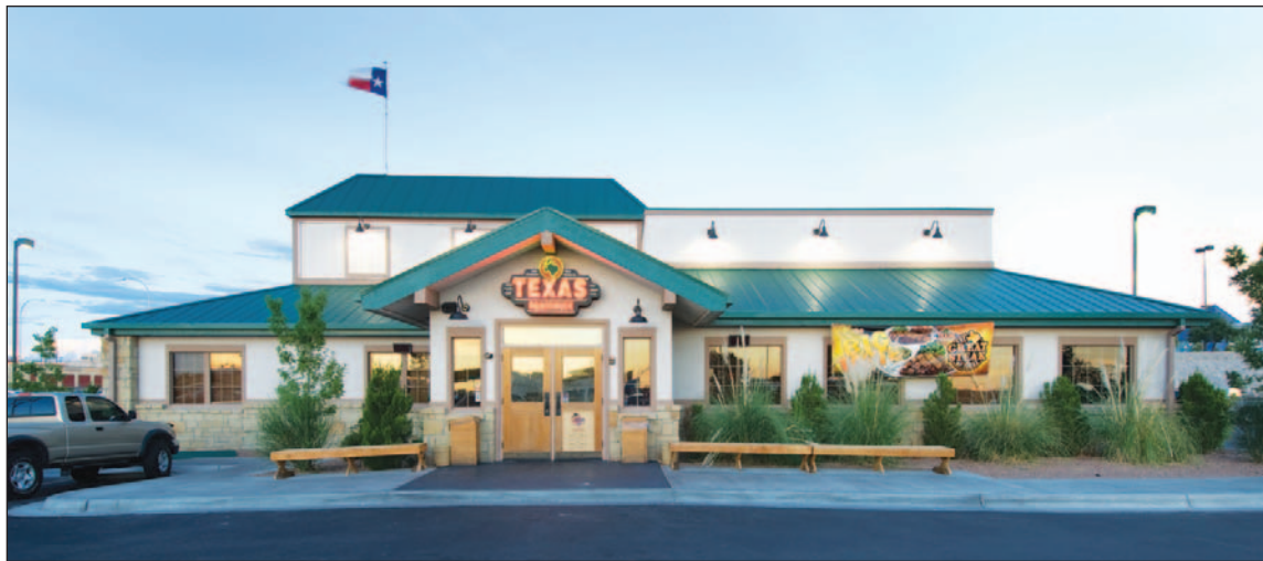
RT Electric provided the lighting services for Texas Roadhouse on Lohman Boulevard.
