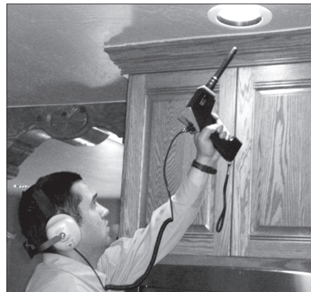
Through Current Safe, a service offered by RT Electric, several tests are conducted to determine if there are any potential electrical hazards, including ultrasonic sound detection, which listens for sparks.
