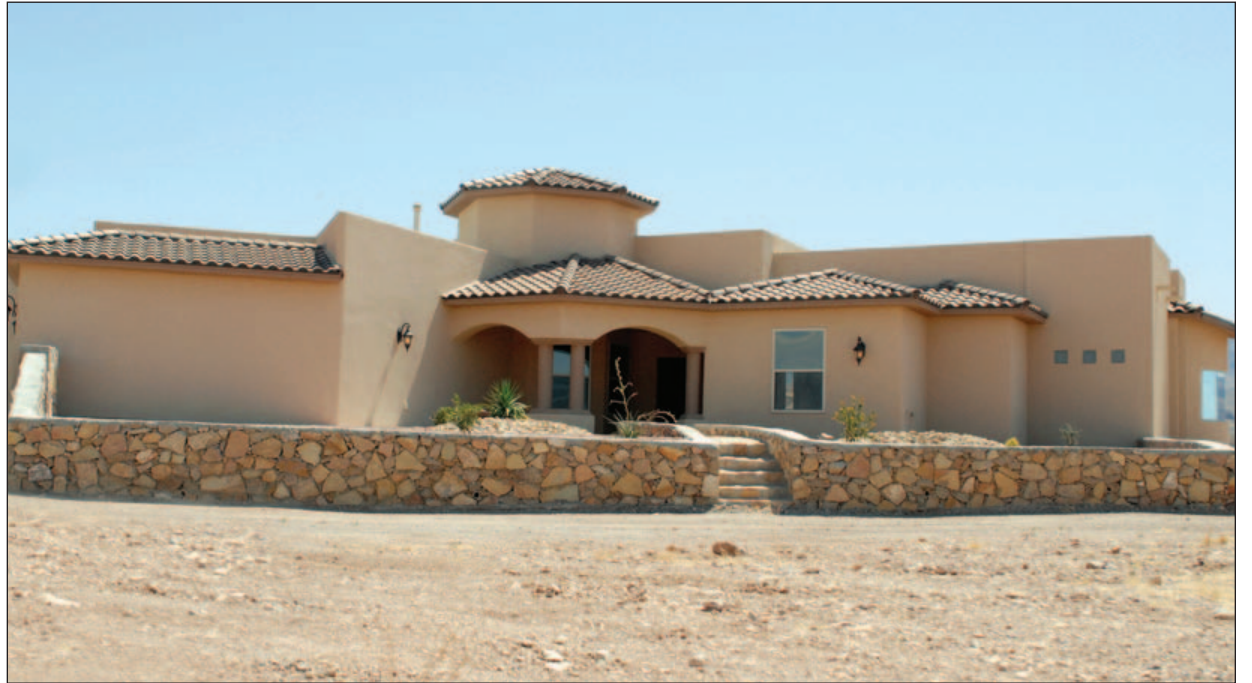
While construction began in 2009, the 3,600-square-foot home at 4131 Camino Bonito was finished in June.
