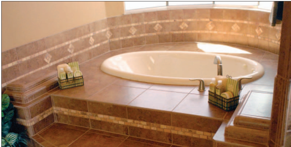
Ceramic and tumbled marble tile surround the jetted bathtub, which is nestled against a bay window.
