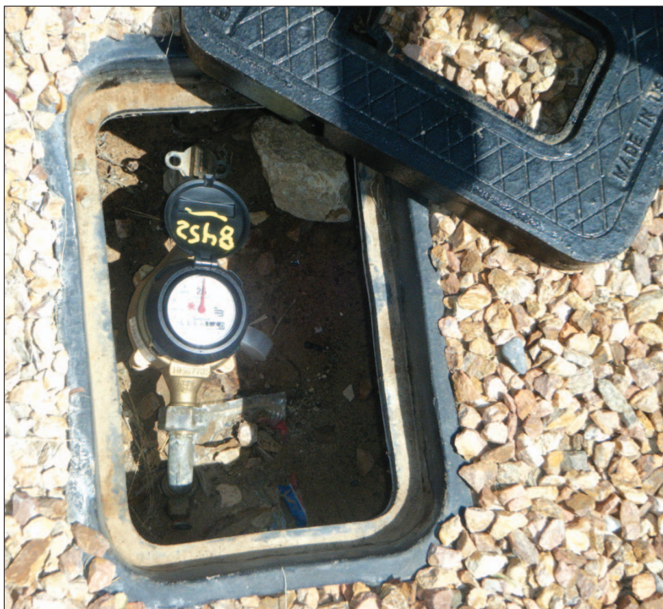
A quick check at your meter dial will let you know if you have unseen leaks on your property.
