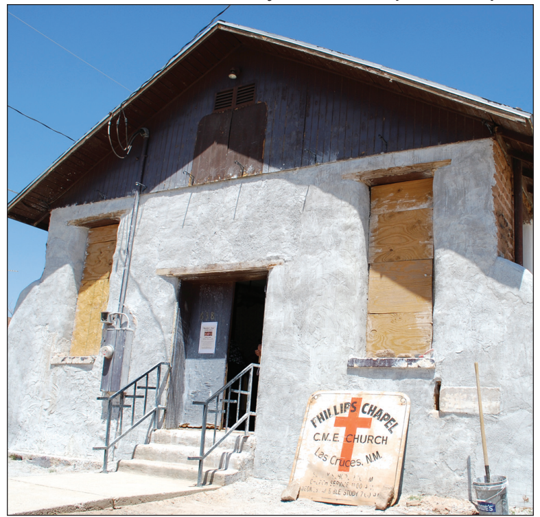
The façade is about 90 percent complete.
