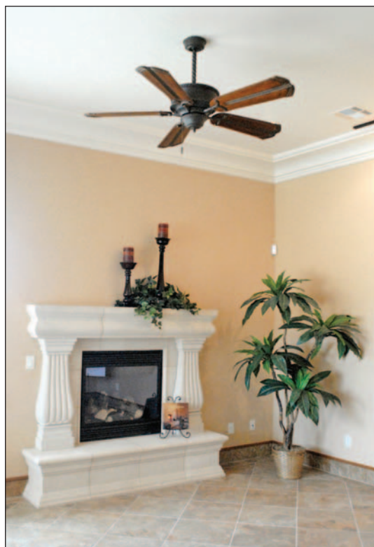
Composite pieces were used to create the fireplace mantel and crown molding.
