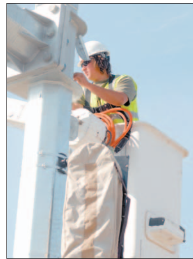
Ryan Chandler checks electrical wiring of a new stoplight.
