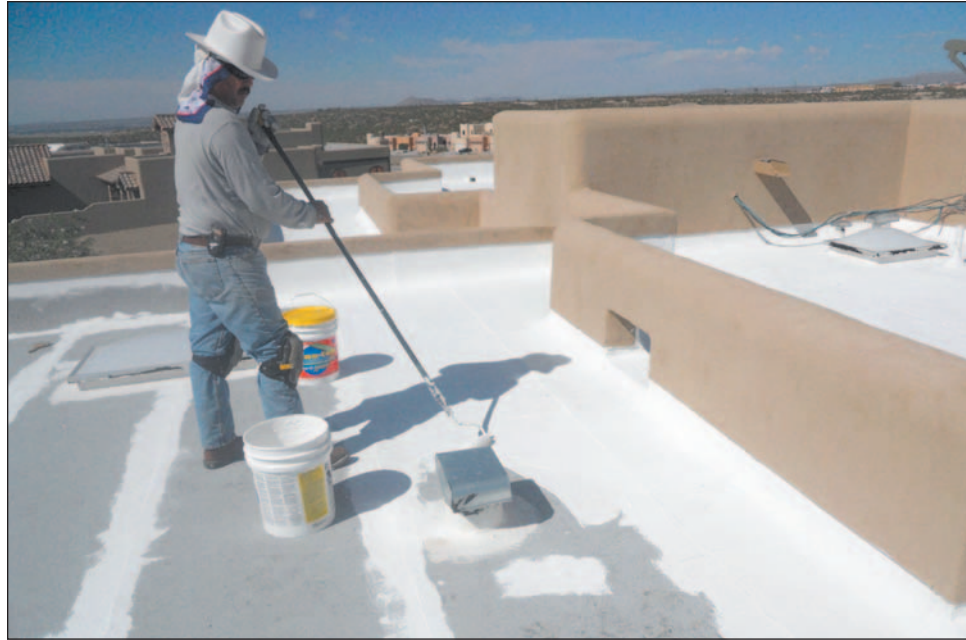
Elastek has taught contractors throughout New Mexico and west Texas how to apply its cool roof, an energy-efficient material, since 2009.
