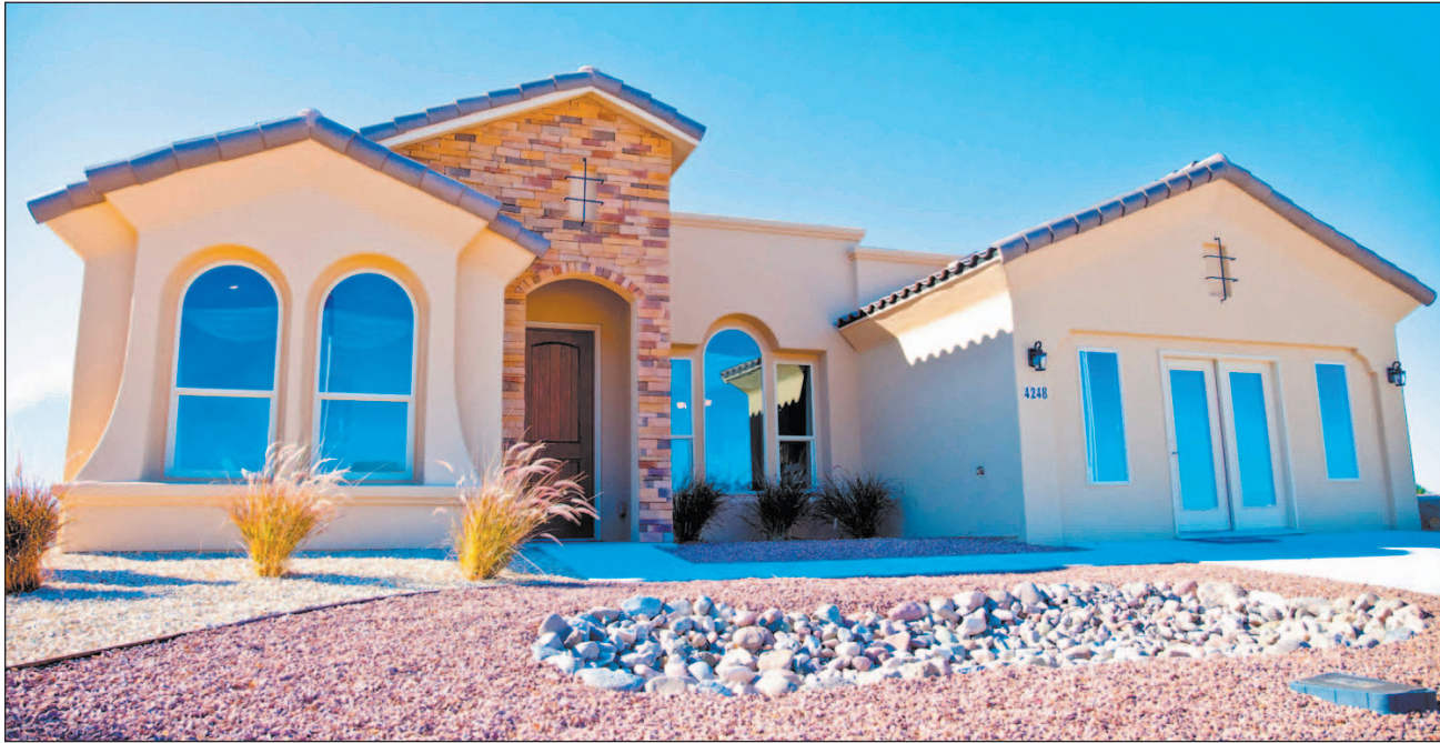
The new model home at 4248 Canterra Arc was completed by Veloz Homes two weeks ago.
