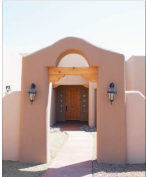
Refined details, such as arches and corbels, can be found in homes built by Robert Hall Homes.
