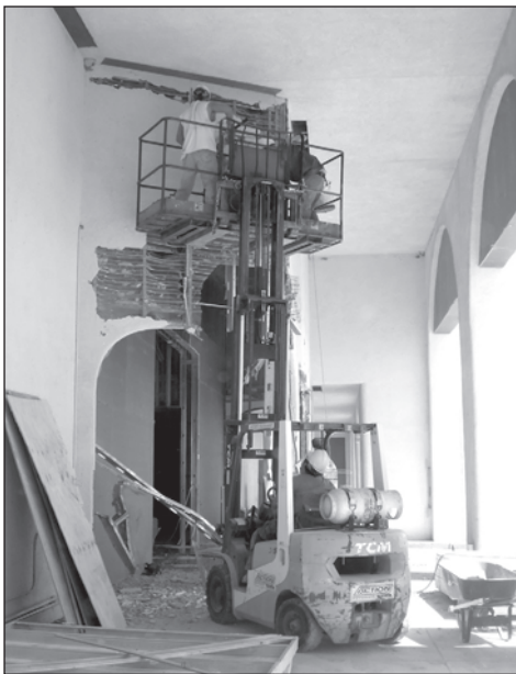
Construction workers hammer out the exterior of Pro's Ranch Market.
