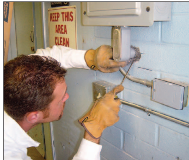
Sealing holes and openings throughout buildings and homes will ensure that pesky insects stay outdoors.
