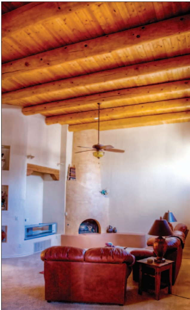
Vigas and wood blanks cover the living room ceiling.
