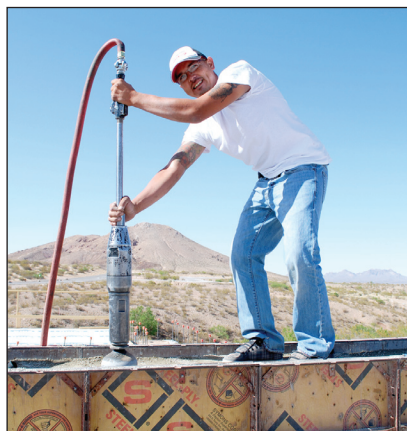
Antonio Rodriguez of Soledad Canyon Earth Builders demonstrates for showcase visitors how the walls are packed down at the home of 7034 Calle Estancias, still under construction.
