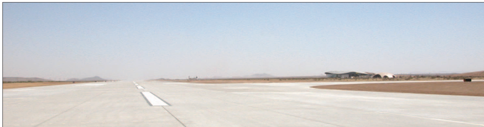
The spaceport's concrete runway is 200 feet wide by 10,000 feet long. It is 42 inches thick with a 14-inch concrete finished surface, which can accommodate almost any manned or unmanned aircraft.
