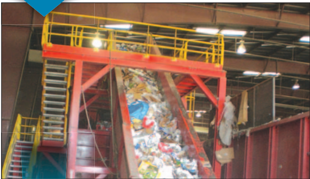
On the conveyor belts, Friedman Recycling processes and separates 25 tons of recyclables an hour.
