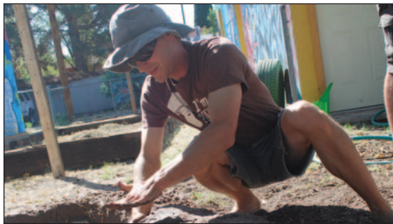
Instructor John Simmons, who taught the cob-building workshop with Lawrence Paxton, pats down the mud and other natural-material mixture to make a bench.
