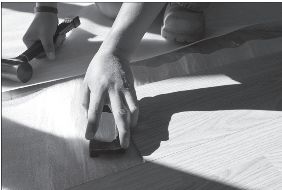
Jason Rouse sets the replacement flooring in place.
